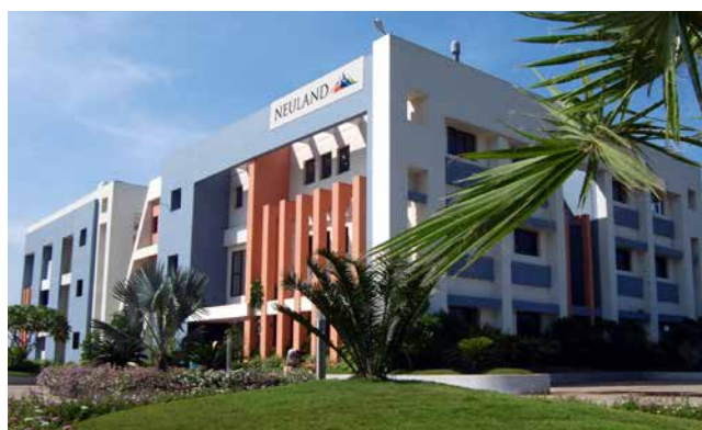
Neuland Laboratories R&D Building, Hyderabad, India
